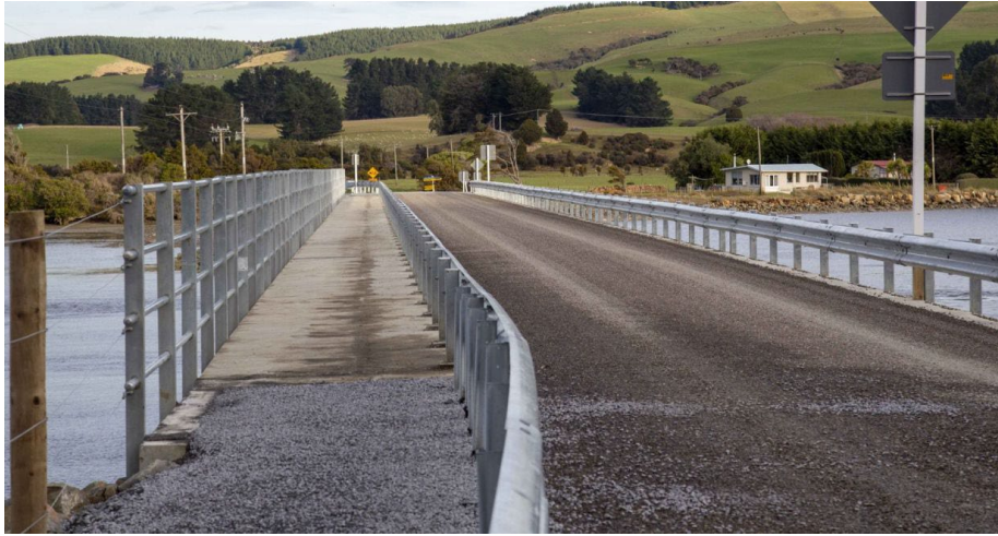
Figure 2-5 The new Hina Hina Bridge
