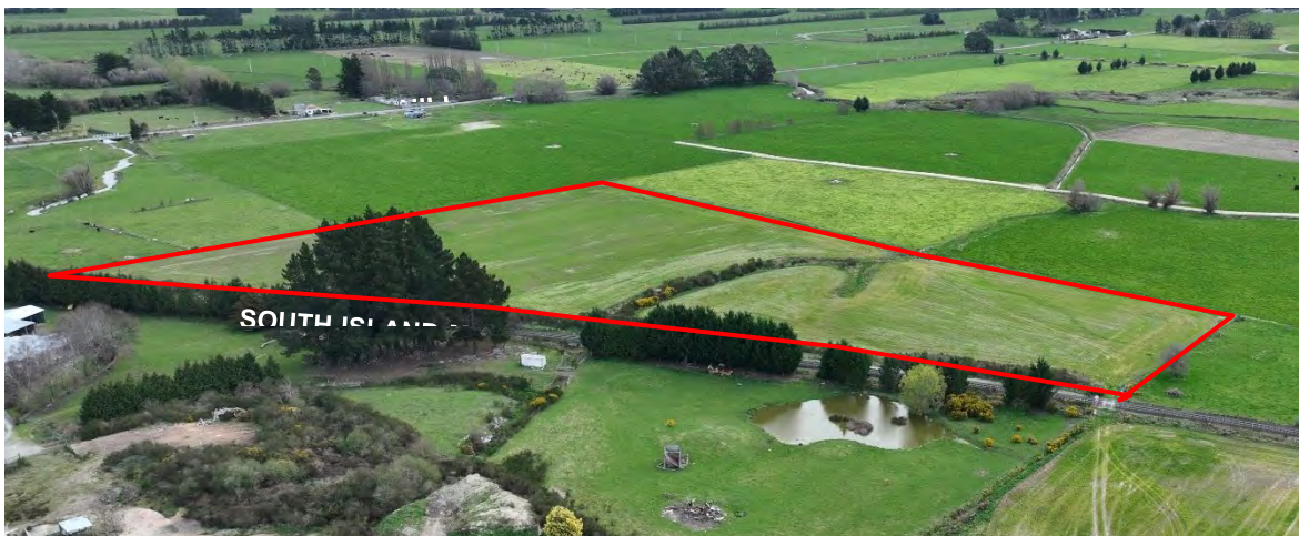
Figure 6-11 Aerial view of Recreation Reserve R69 (boundary indicative only)
