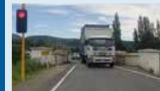
Bridge upgrades ensure our roading network delivers the required level of service.
