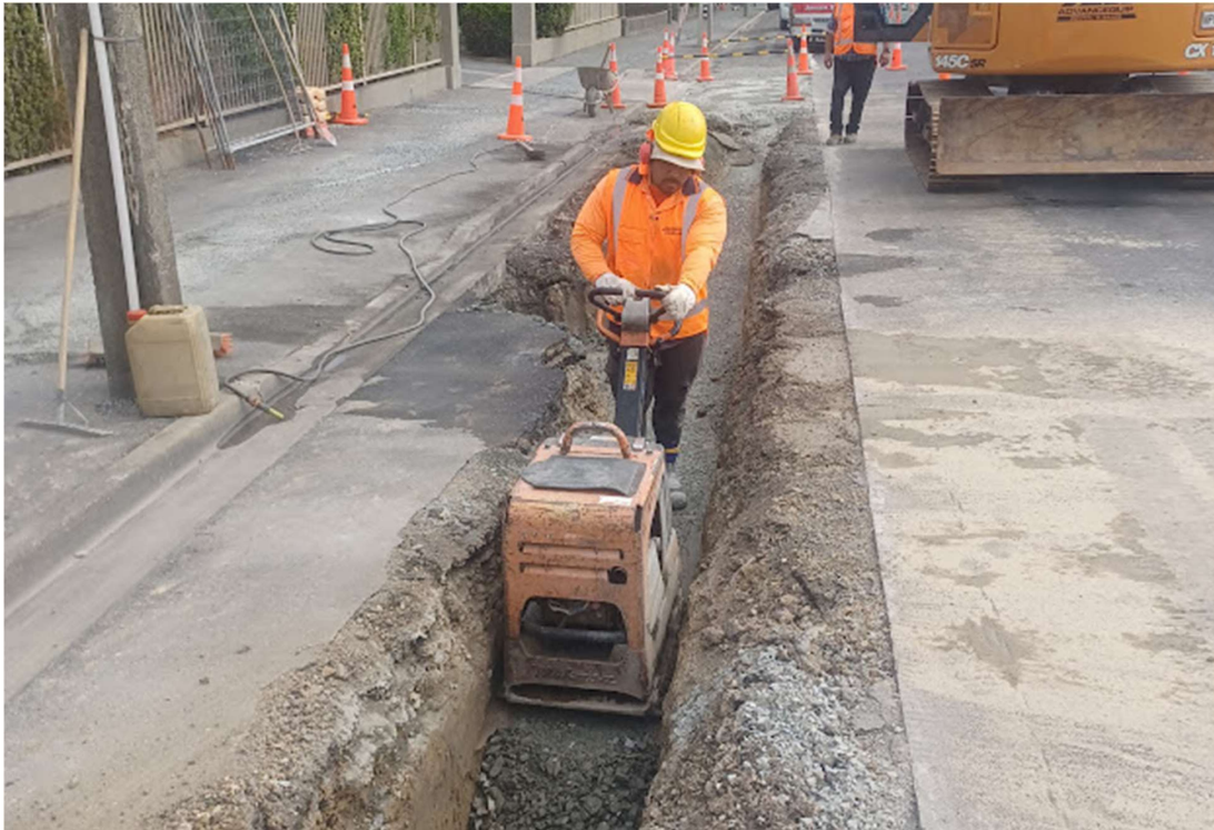
Figure 2 – Milton Mainstreet Additional Ø225 Stormwater pipe - Compacting in layers
