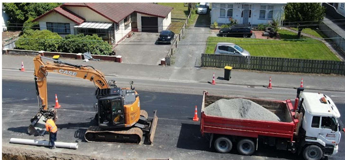
Figure 1 - Milton Mainstreet - Additional Ø225 Stormwater pipe.
