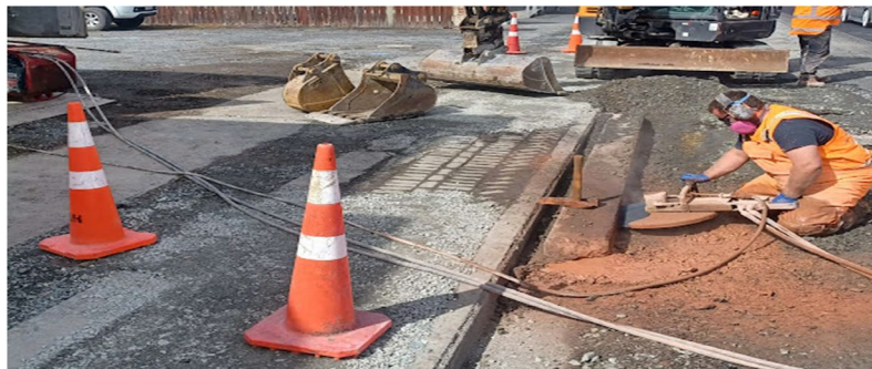
Figure 3 - Slot Crossing being cut at the old Pedestrian Crossing
