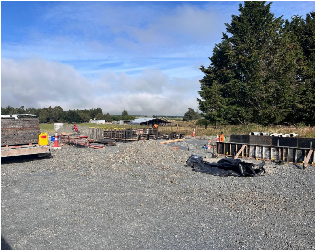
Work underway on the WTP site
