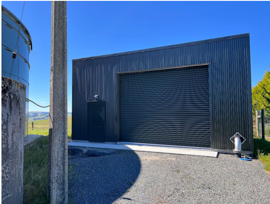
Cairn Road Pump Station
