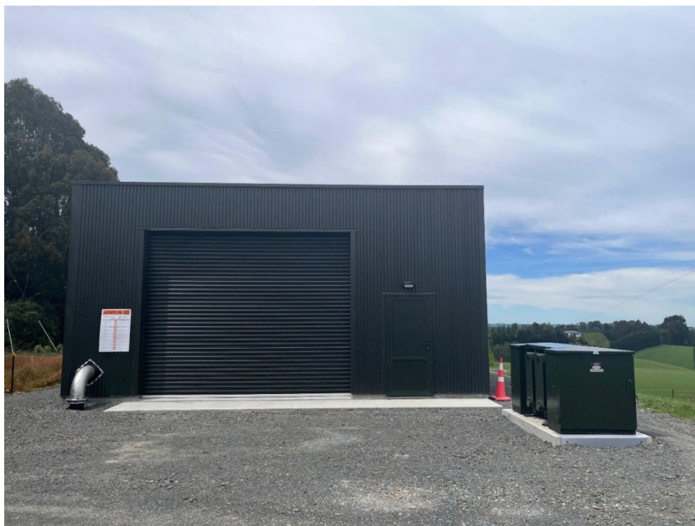
Upper Greenfield Pump Station
