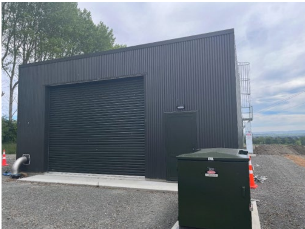
Lower Greenfield Pump Station
