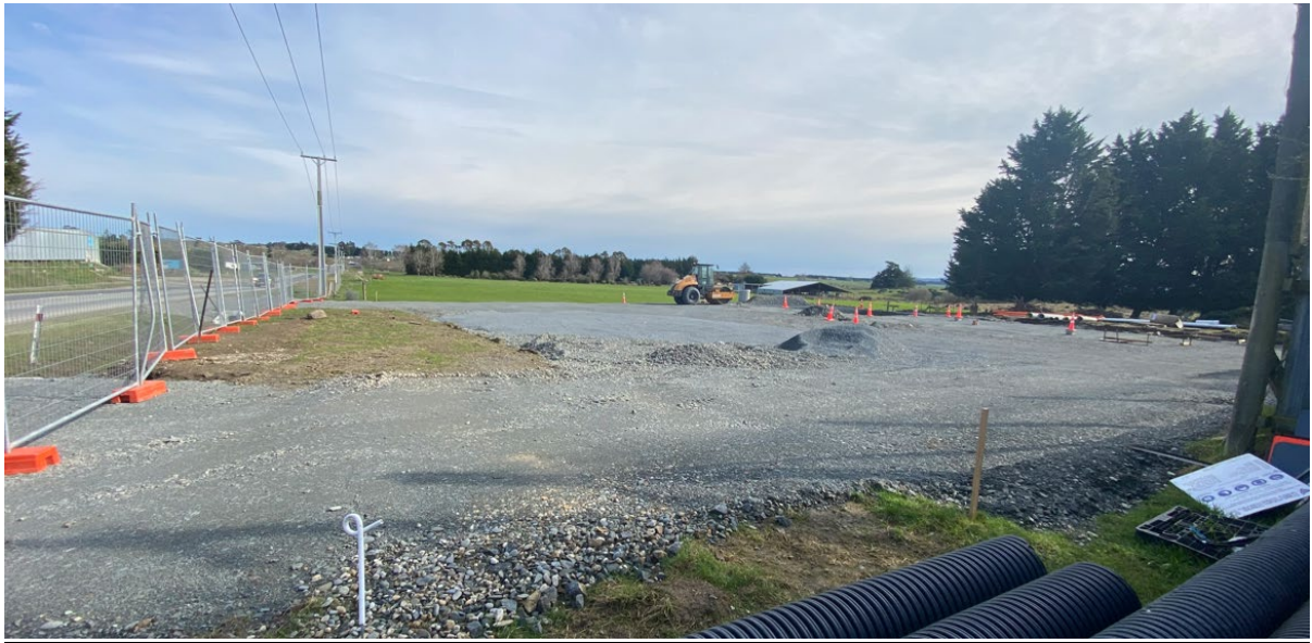
Photo 2 – Work underway on the WTP site
