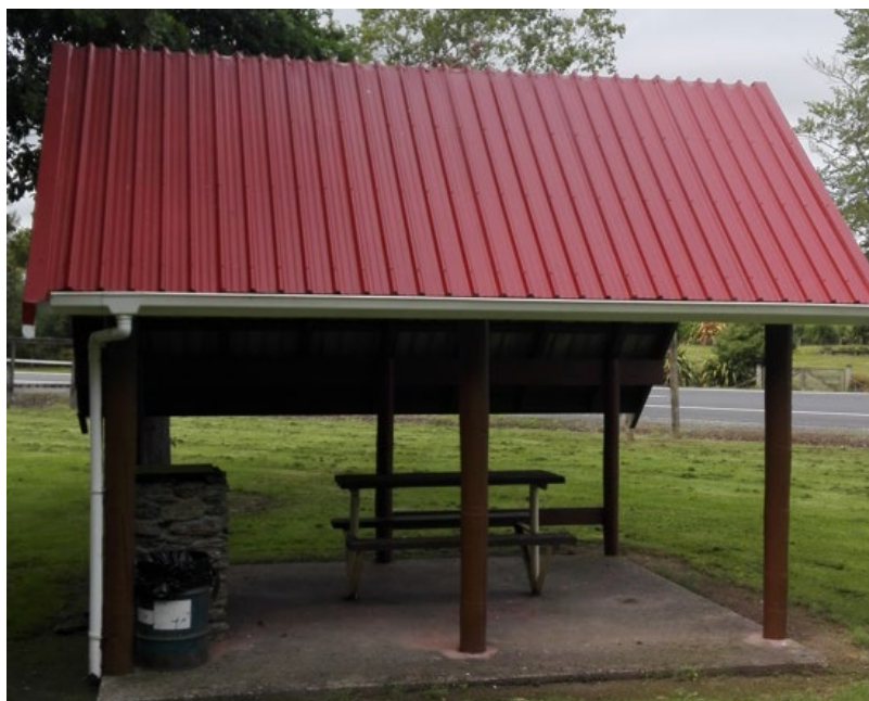
Newly painted Kiosk at Lawrence
