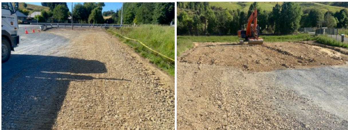
Freedom Camping Site Works
