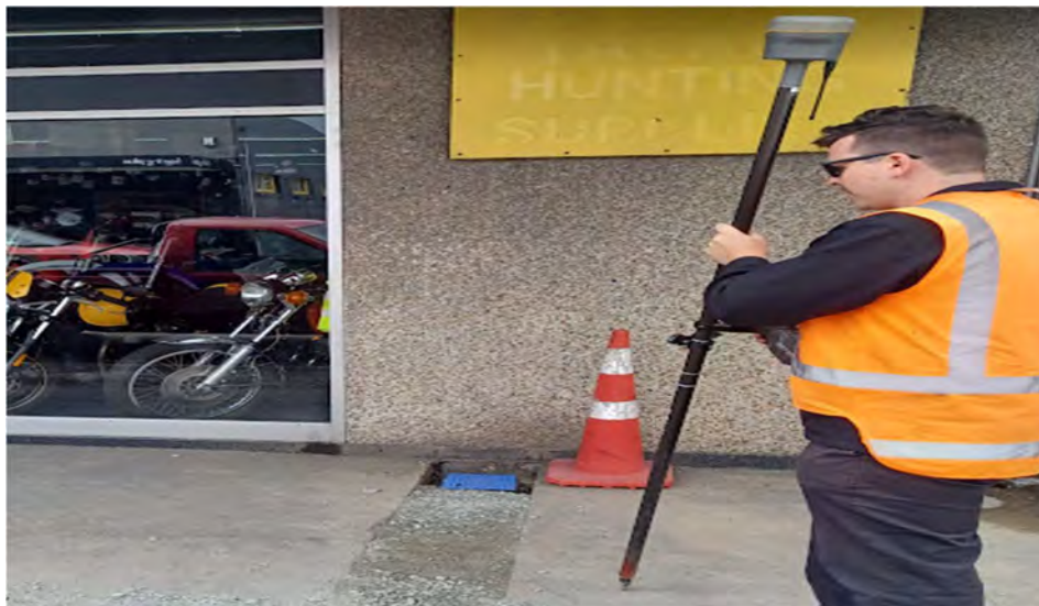
Terramark On-site conducting GPS surveying for as built.
