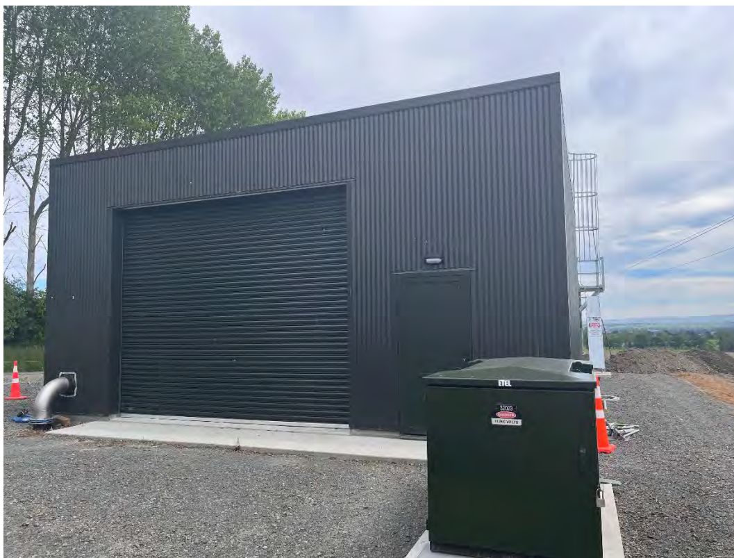
Lower Greenfield Pump Station
