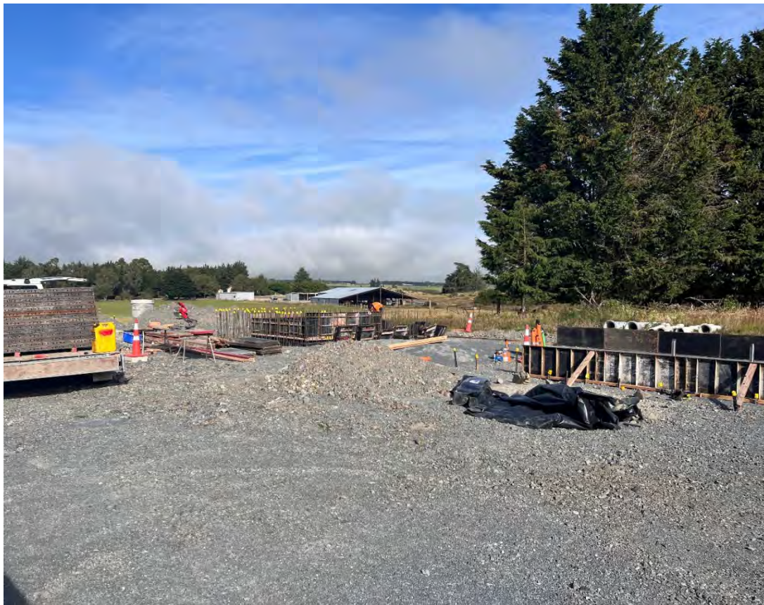
Work underway on the WTP site
