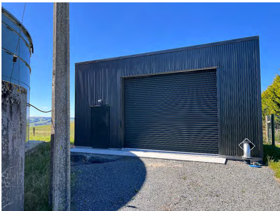
Cairn Road Pump Station
