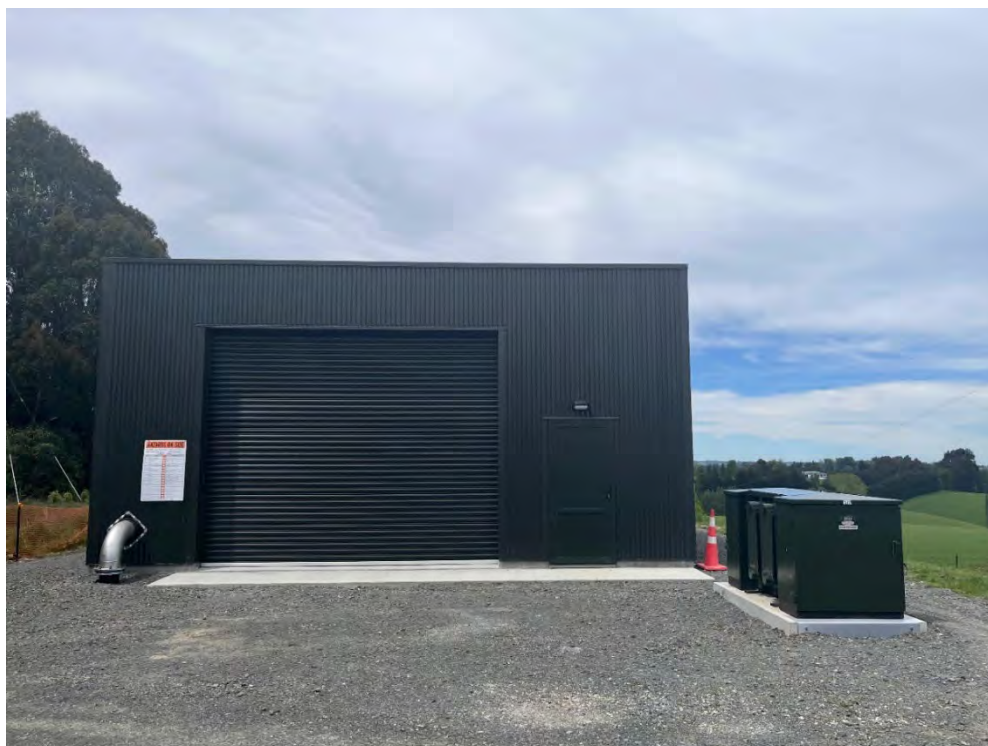
Upper Greenfield Pump Station
