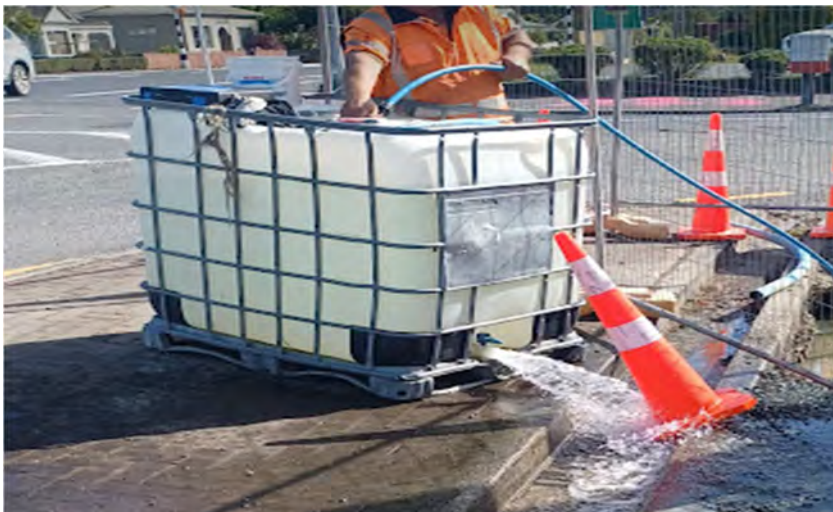
Flushing of the pipeline after pressure testing.
