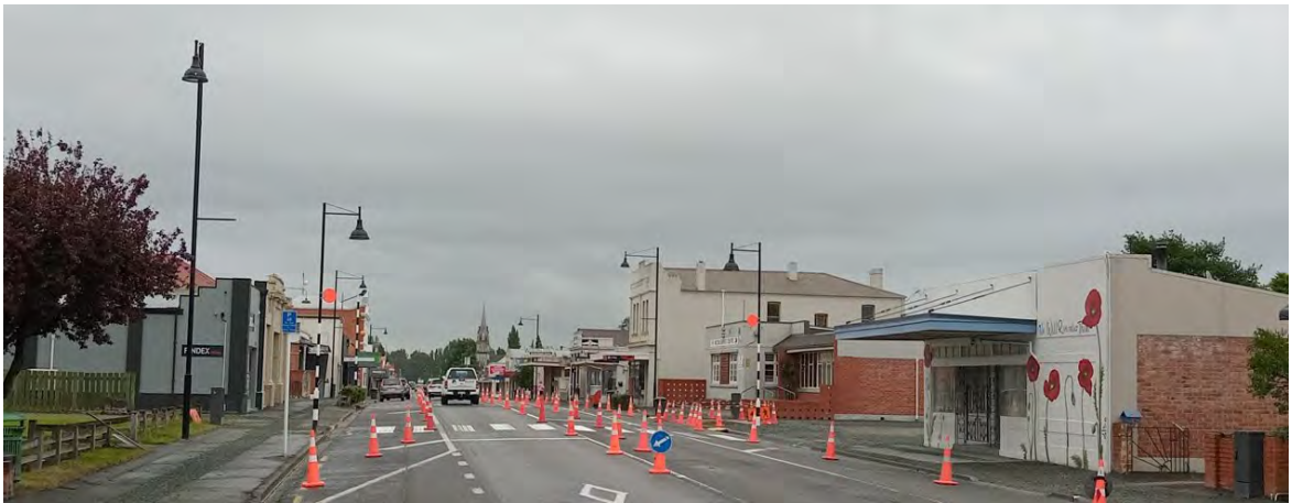
Milton Mainstreet overhead power lines and poles were removed.
