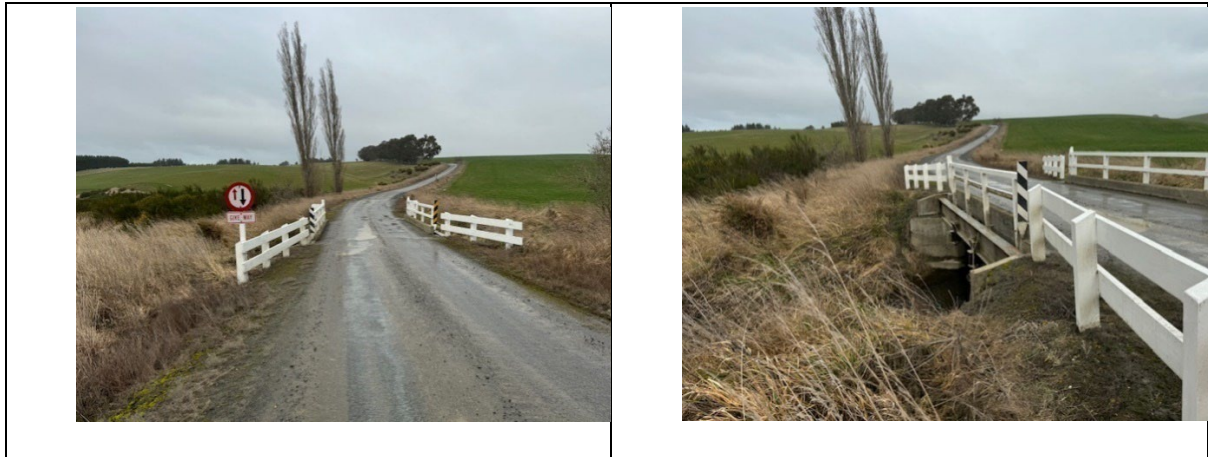
Bridge 121 – Taumata Road - Clinton
