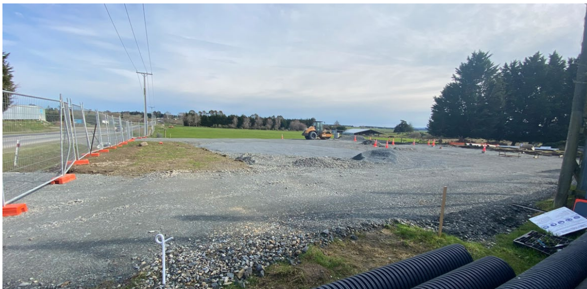
Photo 2 – Work underway on the WTP site
