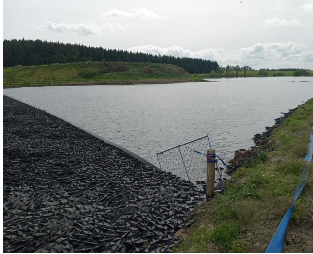
Balclutha Wastewater oxidation pond - hex covers being moved to the correct side of the curtain & in place.
