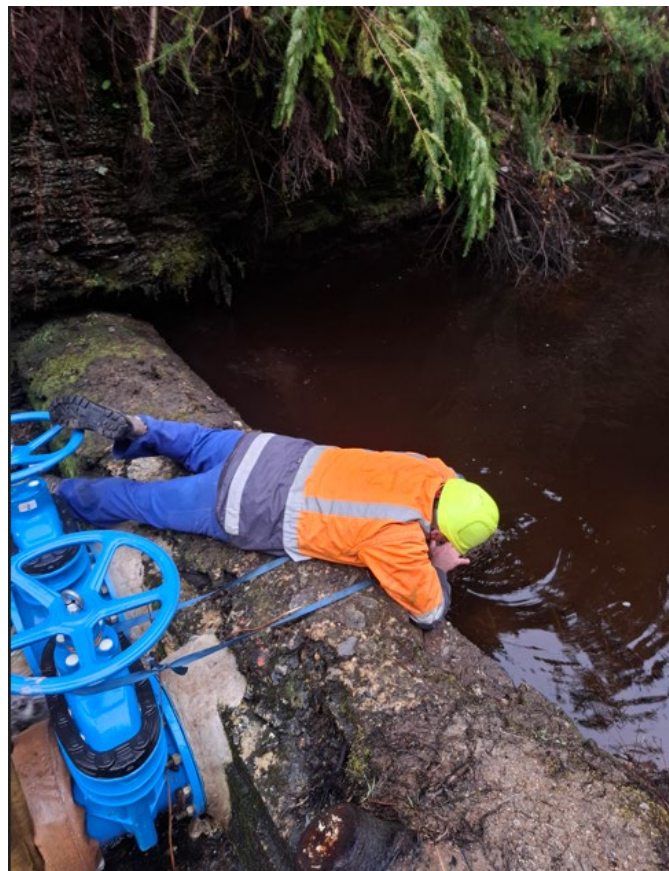
Close up inspection with the siphon valves on the left of the photo
