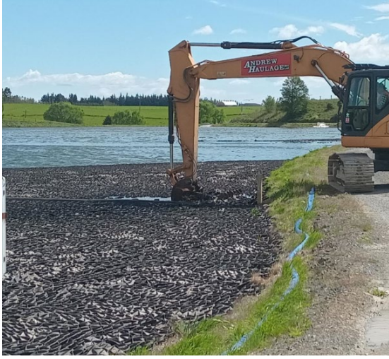
Balclutha Wastewater oxidation pond - hex covers being moved to the correct side of the curtain & in place.
