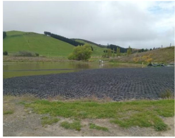
Waiholo Wastewater Treatment Plant – inundated wetlands & still displaced hex covers.
