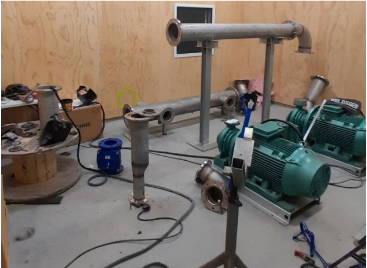
Photo 5 – Cairn Road Pump Station – Progress on Pipework
