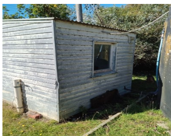
Mt Mistake Pump Station Exterior
