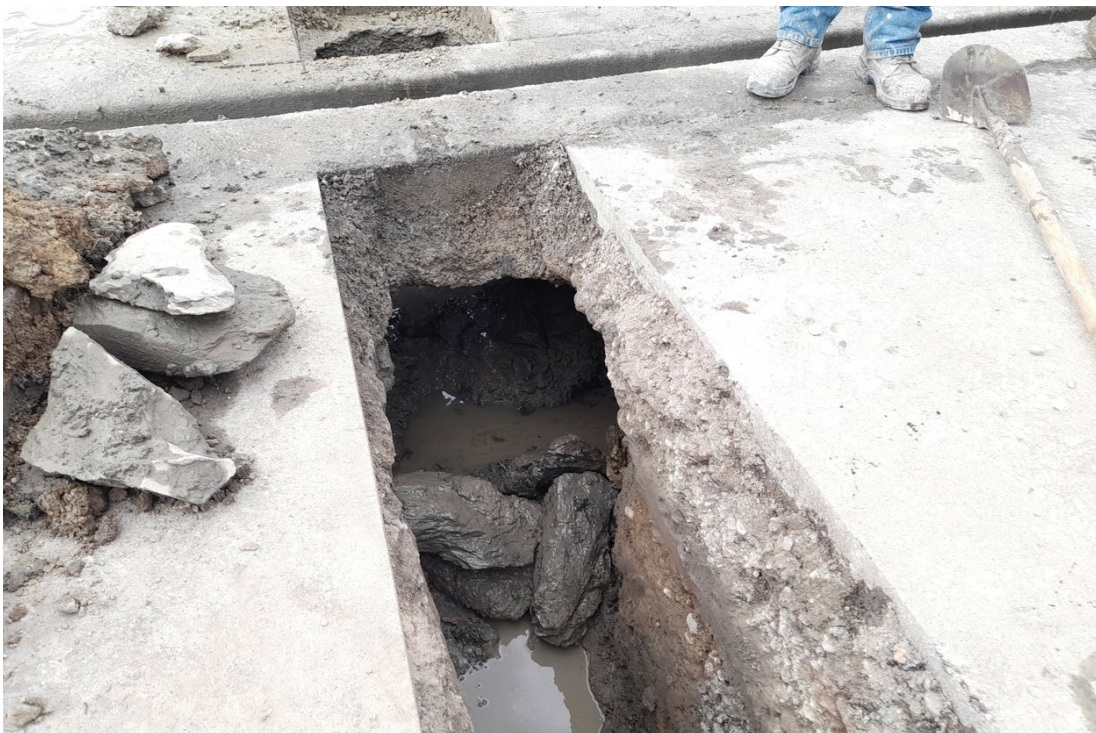
Abercrombie St. - Blue stone Culvert Pre 1900 Feature
