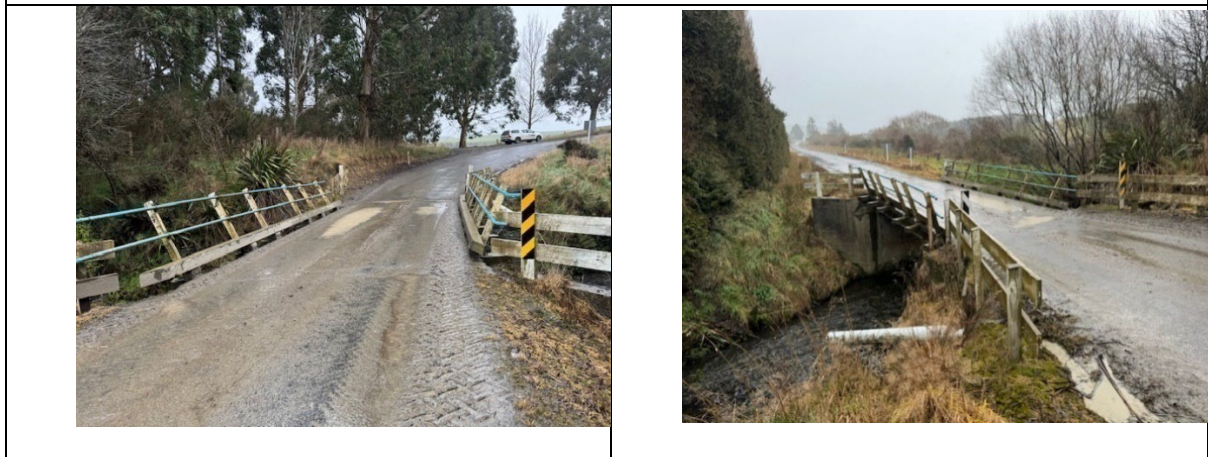
Bridge 147 – Slopedown Road - Catlins
