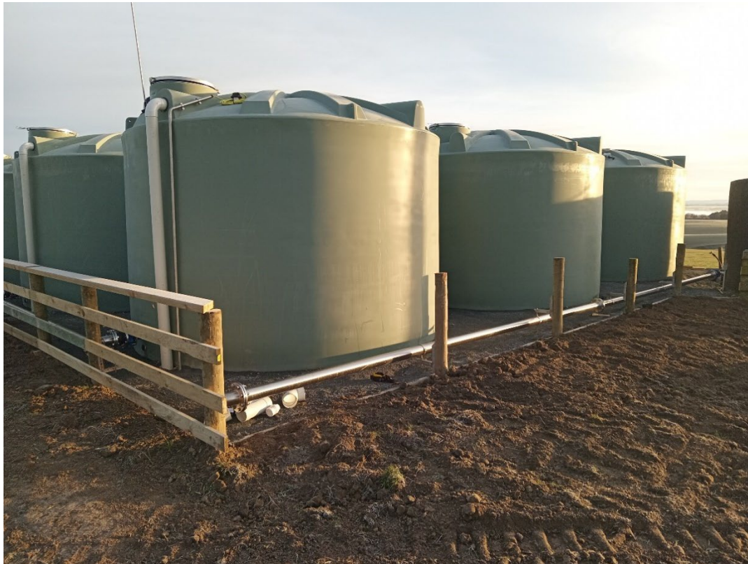
30m3 New Plastic Tank Farm Reservoir
