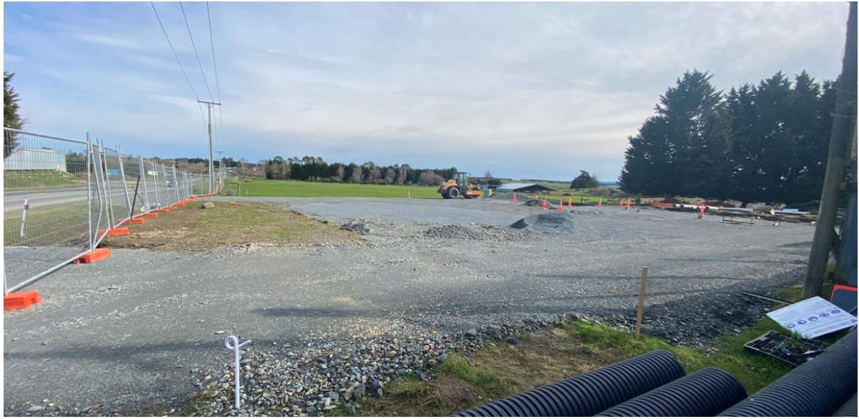
Photo 2 – Work underway on the WTP site
