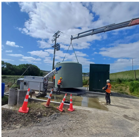
Inlet screen tank setting for Balclutha WWTP Inlet
