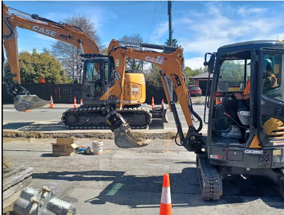
Milton Union Street – Machinery used on the Stormwater Pipeline Extension.
