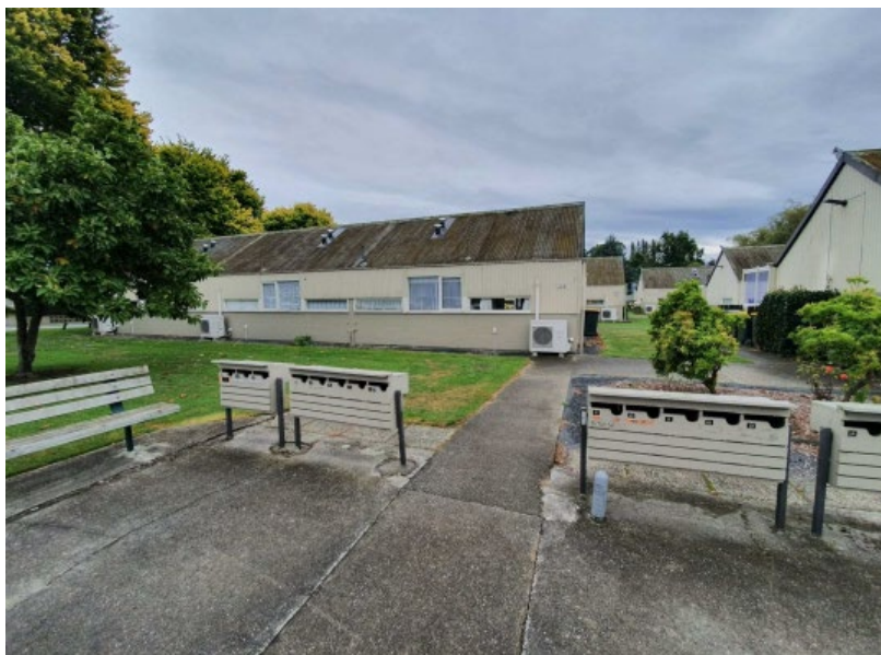
Figure 1. Naish Courts Community Housing Units (64 Charlotte Street, Balclutha)
