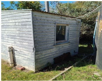
Mt Mistake Pump Station Exterior
