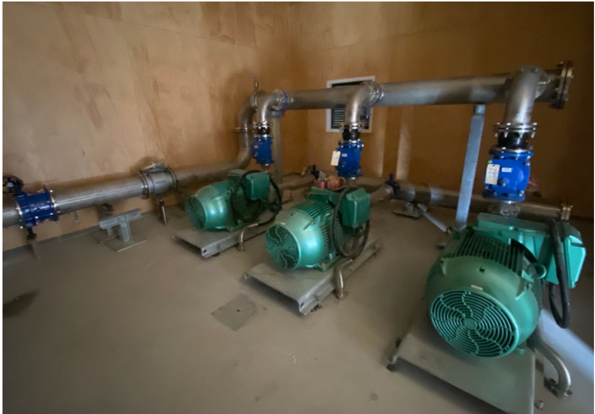
Photo 4 – Upper Greenfield Pump Station – progress on the pipework
