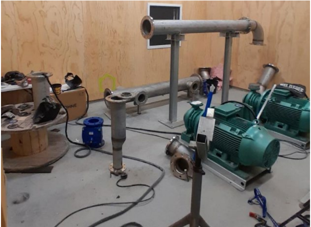
Photo 5 – Cairn Road Pump Station – Progress on Pipework
