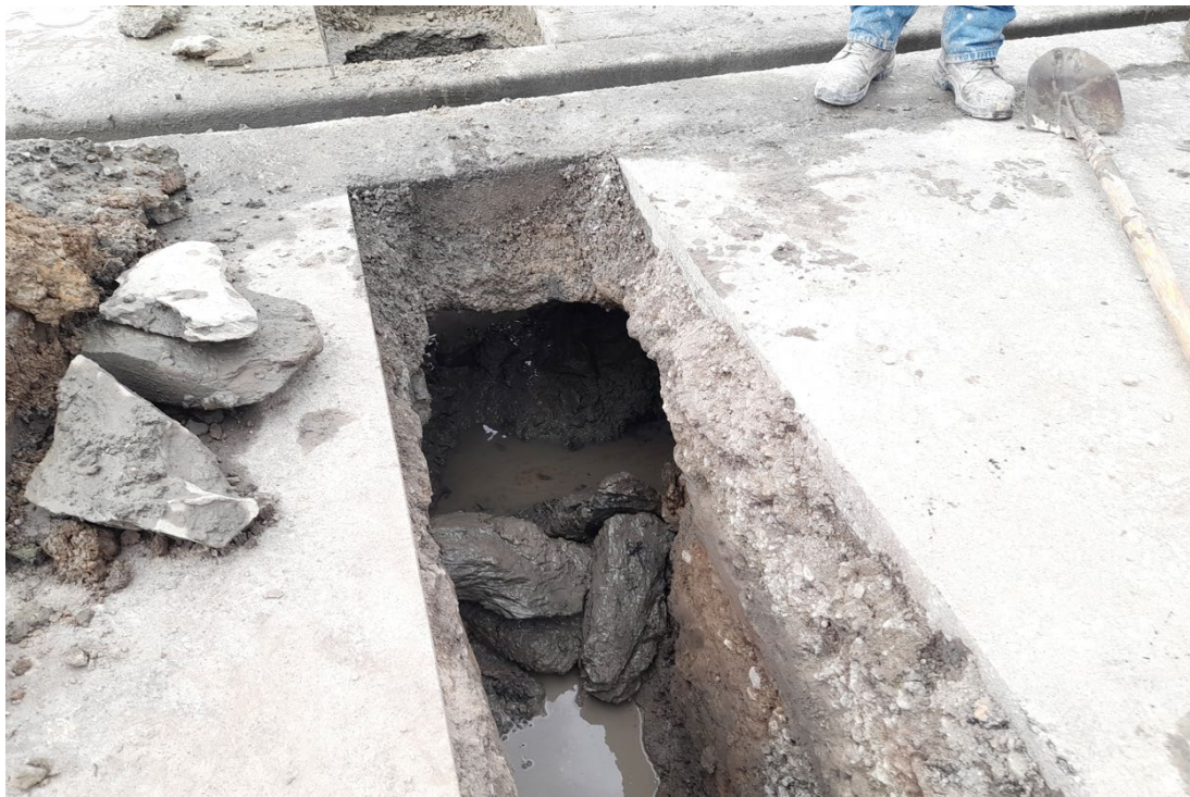
Abercrombie St. - Blue stone Culvert Pre 1900 Feature
