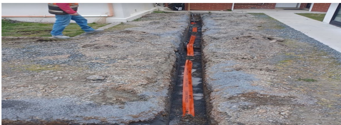
Inside property connection with power cable installed under crusher dust and warning tape on Union Street.
