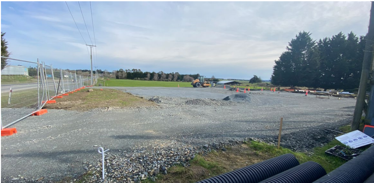
Photo 2 – Work underway on the Water Treatment Plant site
