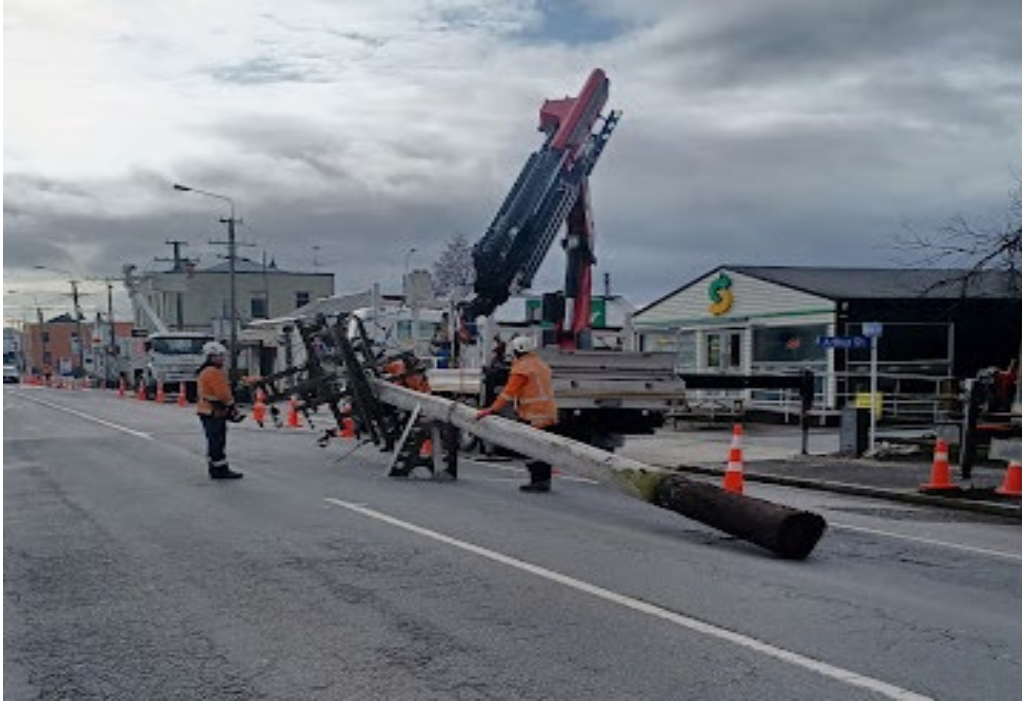
Pole removal from Union St
