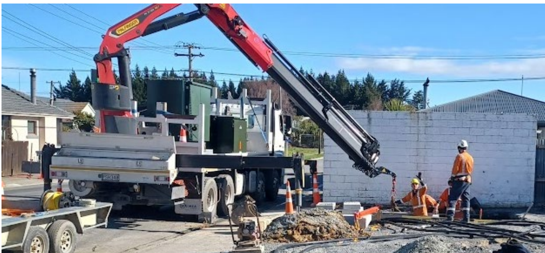
Installation of the second transformer and ring mains on Gray Street
