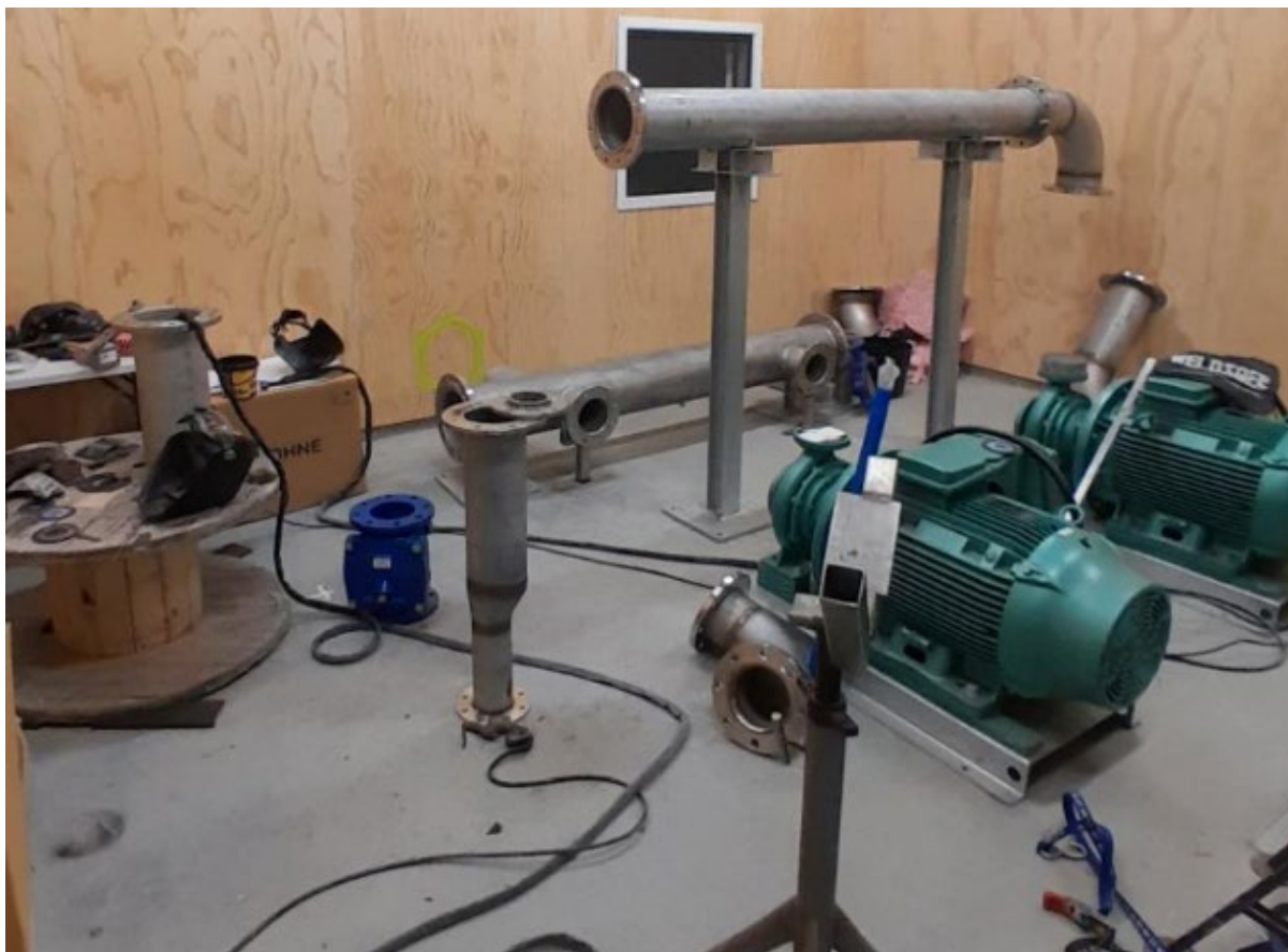
Photo 7 – Cairn Road Pump Station – Progress on Pipework (beginning of Sept)
