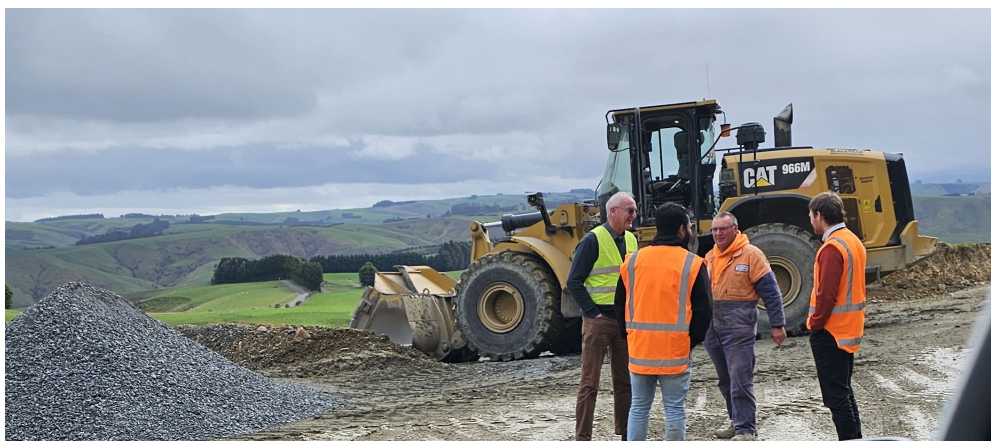
Transportation Team Visit to Lyders Quarry to check condition of metal.
