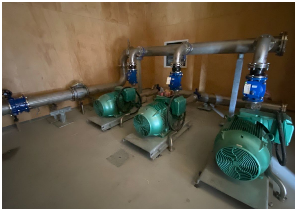
Photo 5 – Upper Greenfield Pump Station – Progress on Pipework
