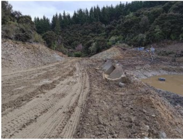
Photo 1: Upstream face of dam looking west
