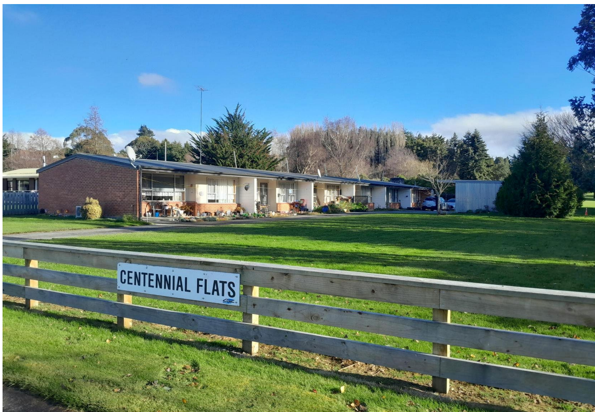
Figure 1. Clinton Community Housing Units
