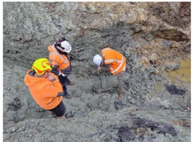
Photo 4: Hand excavations around low-level conduit
