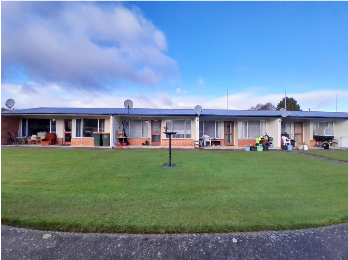
Figure 2 Owaka Community Housing Units
