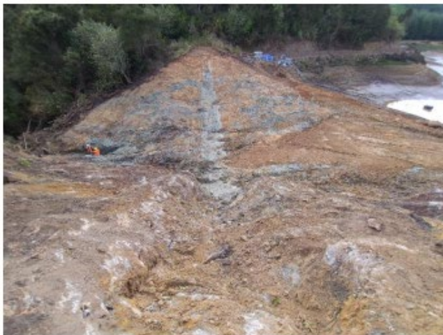
Photo 3: View along excavation from left abutment
