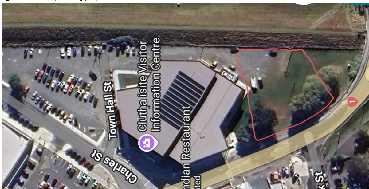
Figure 1 - Aerial photo of proposed location
