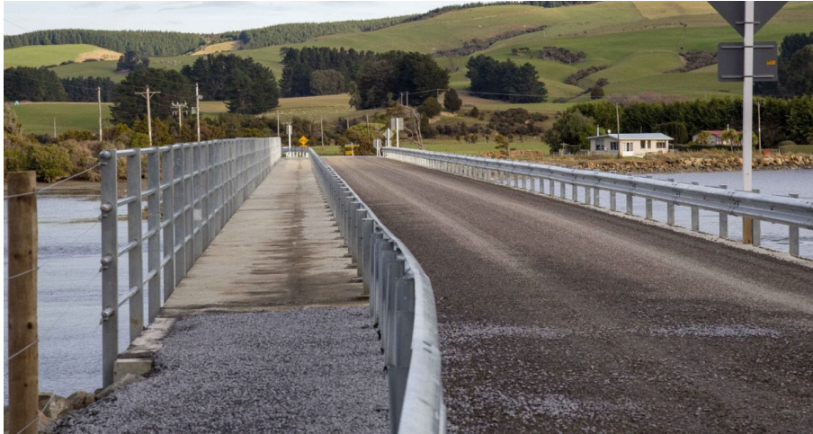
Figure 2-5 The new Hina Hina Bridge
